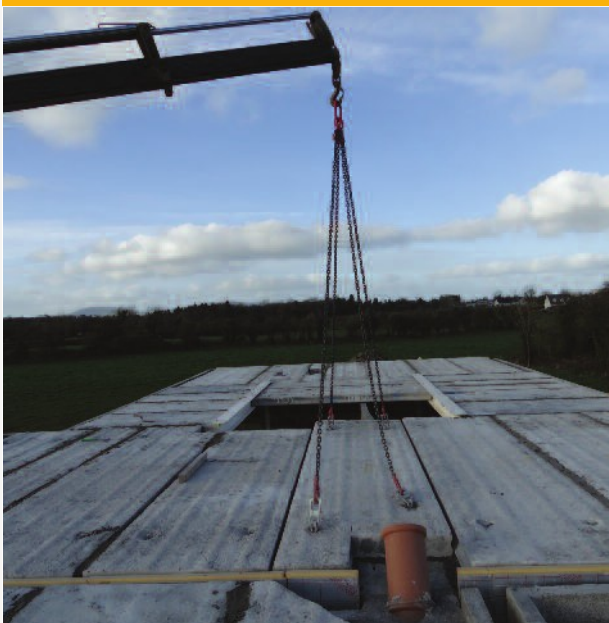
Installation with crane
