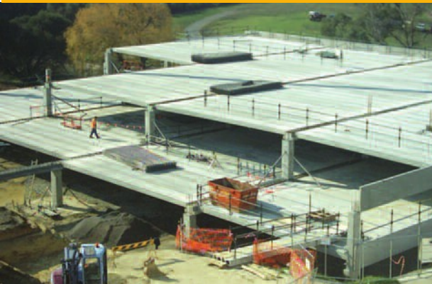
Slab installation
