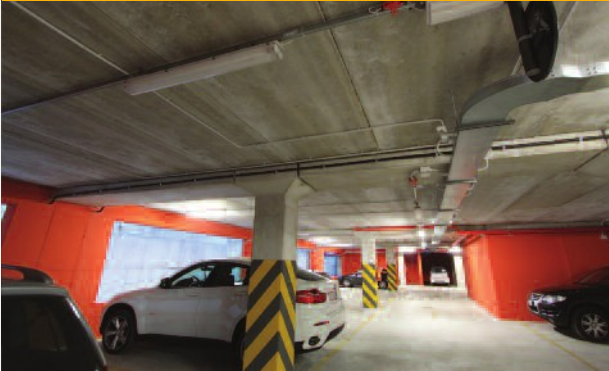
Car park soffit view
