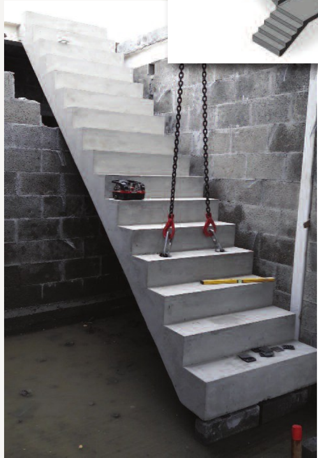
Example of stairs installation
